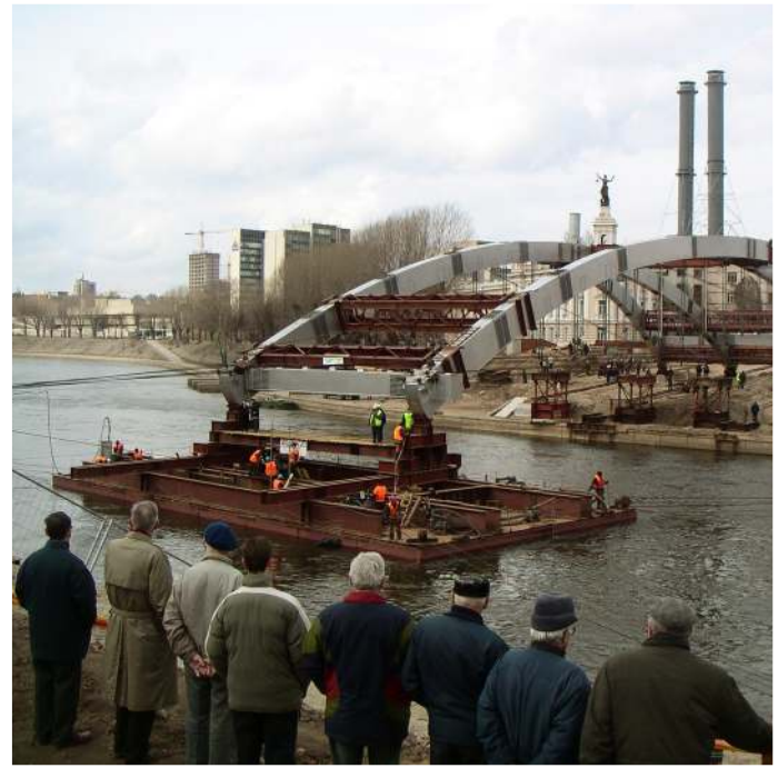
Construction of Mindaugas bridge (Photo: Vilnius OTRA)
